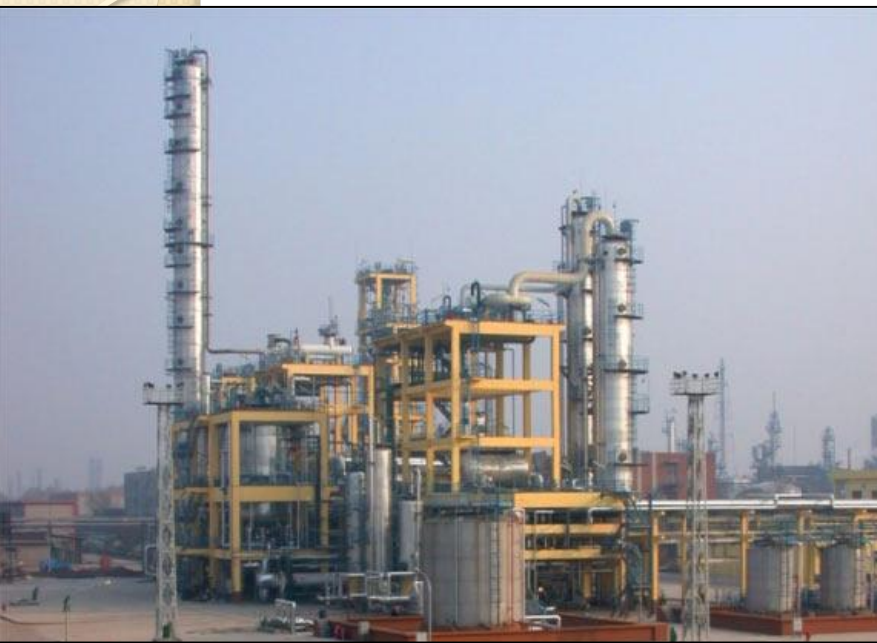
2-Ethylhexanol plant built by Sinopec Qilu Petrochemical Co. Ltd., China, employing the LP Oxo SM Process
