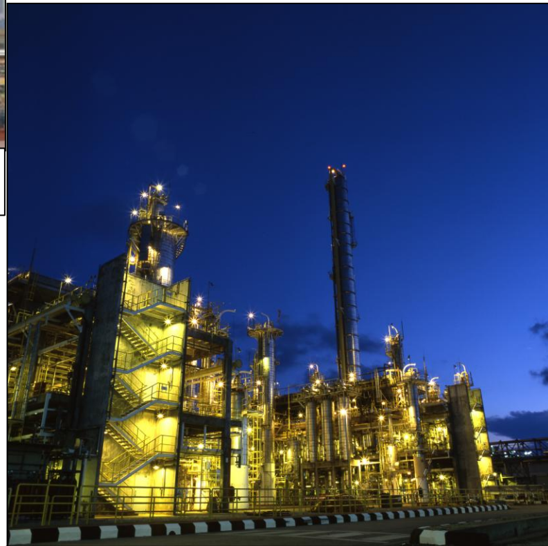
Oxo/Syngas complex at the Verbund site Kuantan, Malaysia
