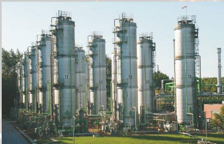
Oxidation units in which cumene hydroperoxide is produced
